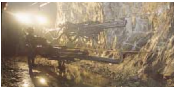
UNDERGROUND DRILLING AT OBUASI
